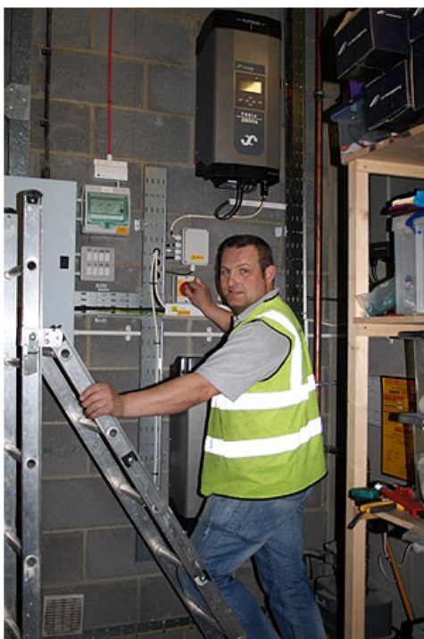
Project manager Brian Hamilton starts-up our solar generated electricity.
